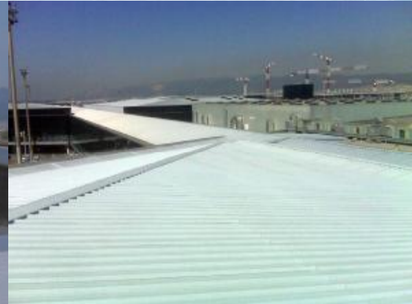
Barcelona Airport Refurbishment of pre-boarding areas Impermax Plus System Arq. Ineco Ing.
